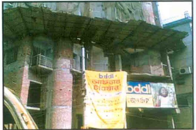
Commercial Building Project
